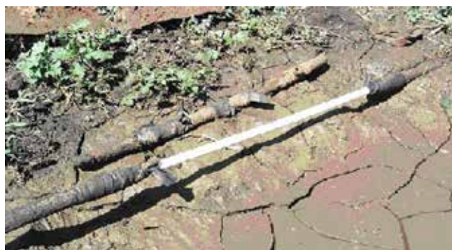
FIGURE 3–12 Leaked pipe repaired with bicycle tubing
