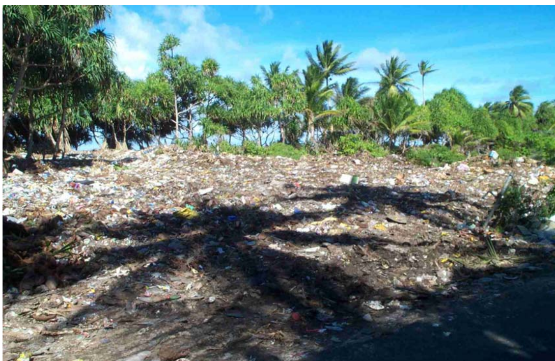
Figure 1. Fongafale waste collection site (old borrow pit) desperately requires capping material (some 2500 m 3 of general-purpose fill is presently required to cap the landfill to 0.4 m).
