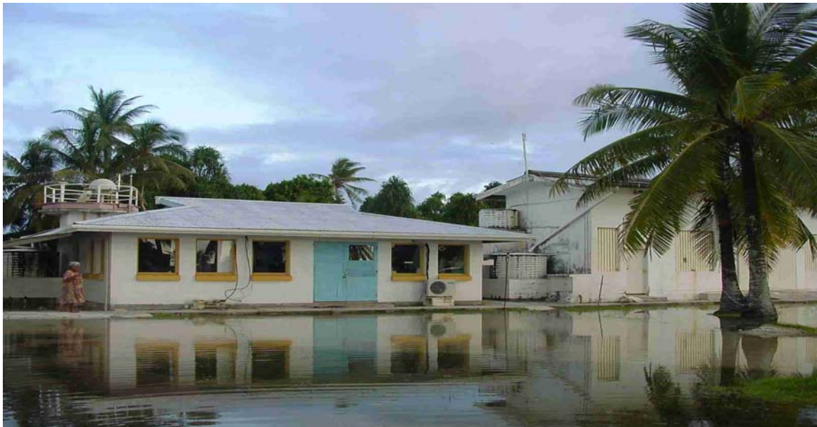
Figure 2. Funafuti Meteorological Office, inundated with seawater during spring tide conditions (tides > 2.8 m), the western side of the airstrip requires some 7500 m 3 of fill to raise the surrounding area 0.3 m.
