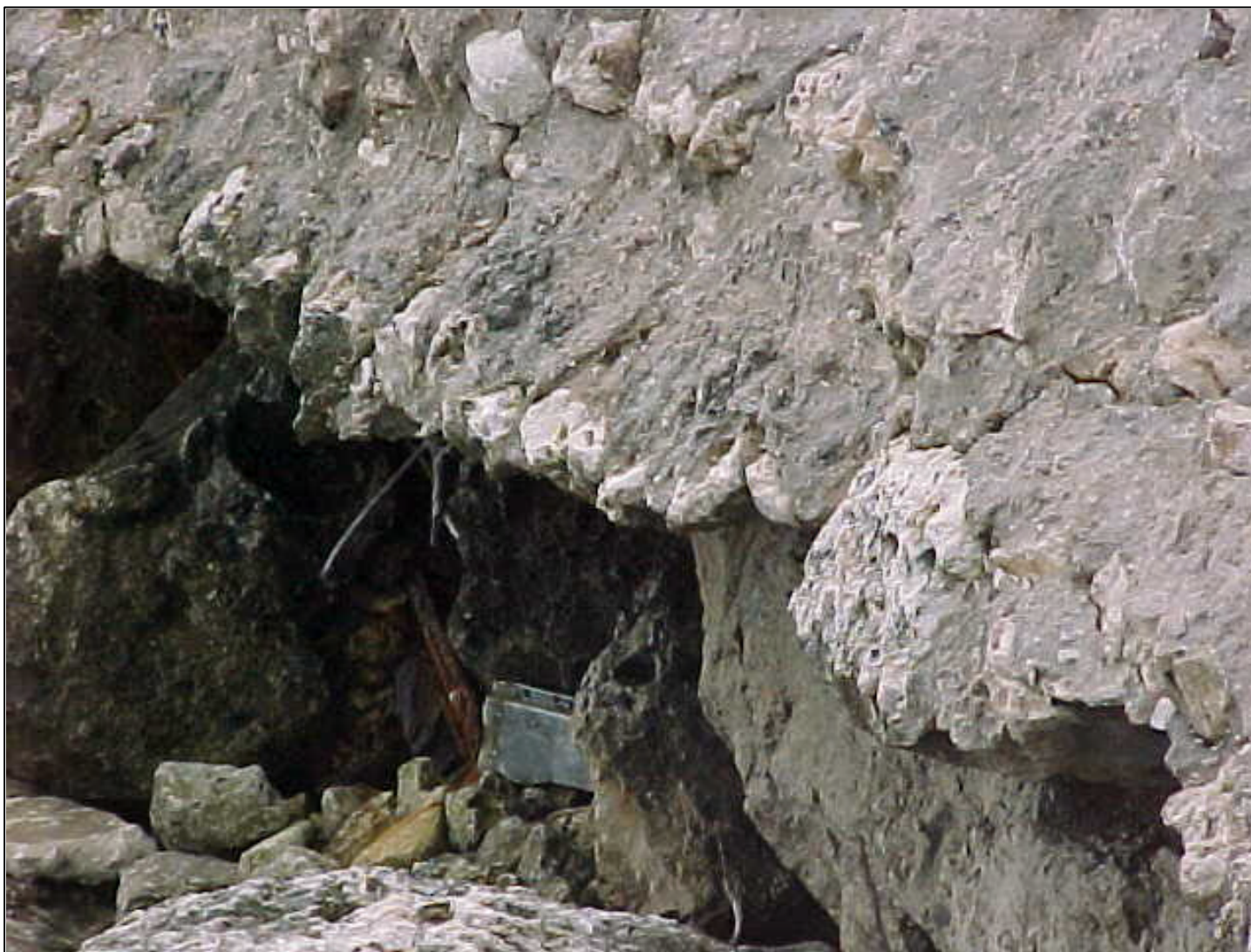
Figure 19. Details of the scoured western section of the scoured retaining wall.
