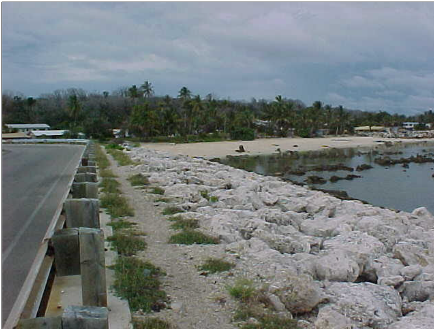
Figure 30. View looking north-northeast showing the rip-rap revetment protecting the airport and coastal roadway. Note limestone pinnacles in the surf zone (to the right).
