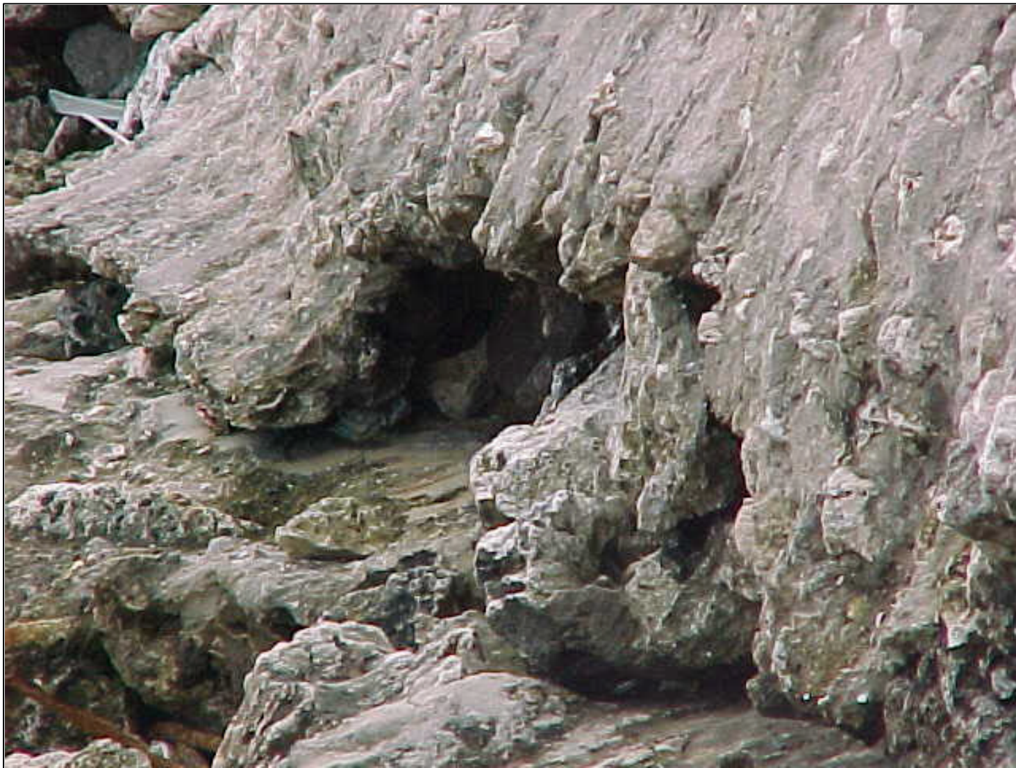
Figure 22. Scouring and removal of wall aggregate due to wave action and abrasion.
