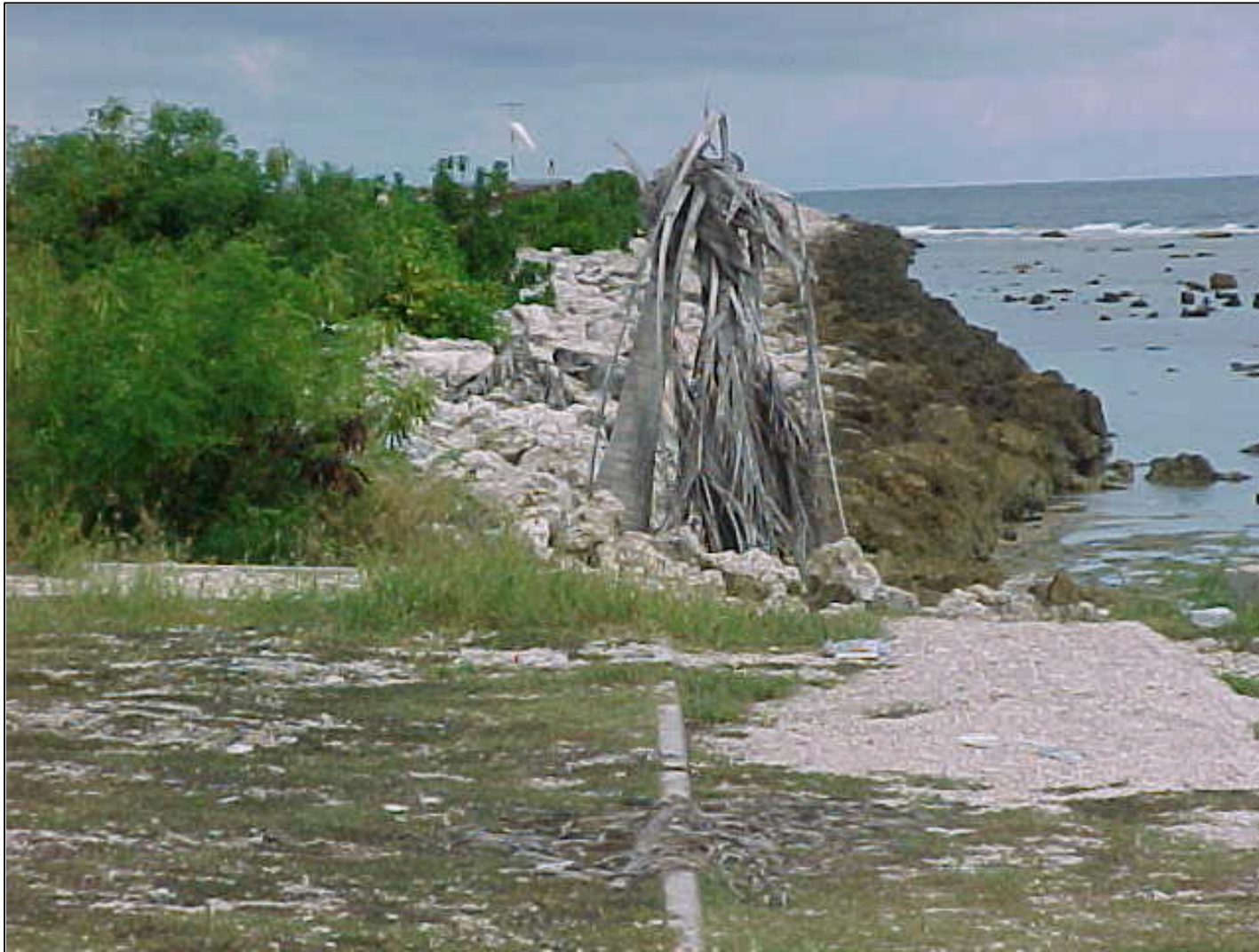
Figure 14. Details of the fill protection using rip-rap revetment.
