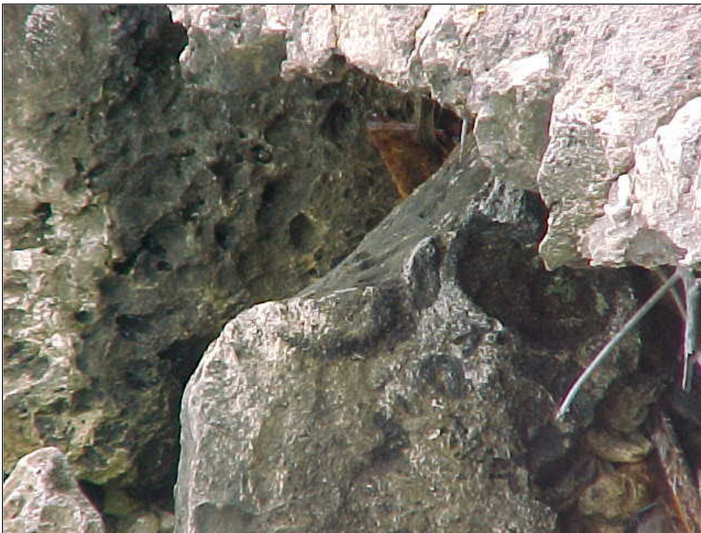
Figure 20. Large cavities at the base of the scoured retaining wall.
