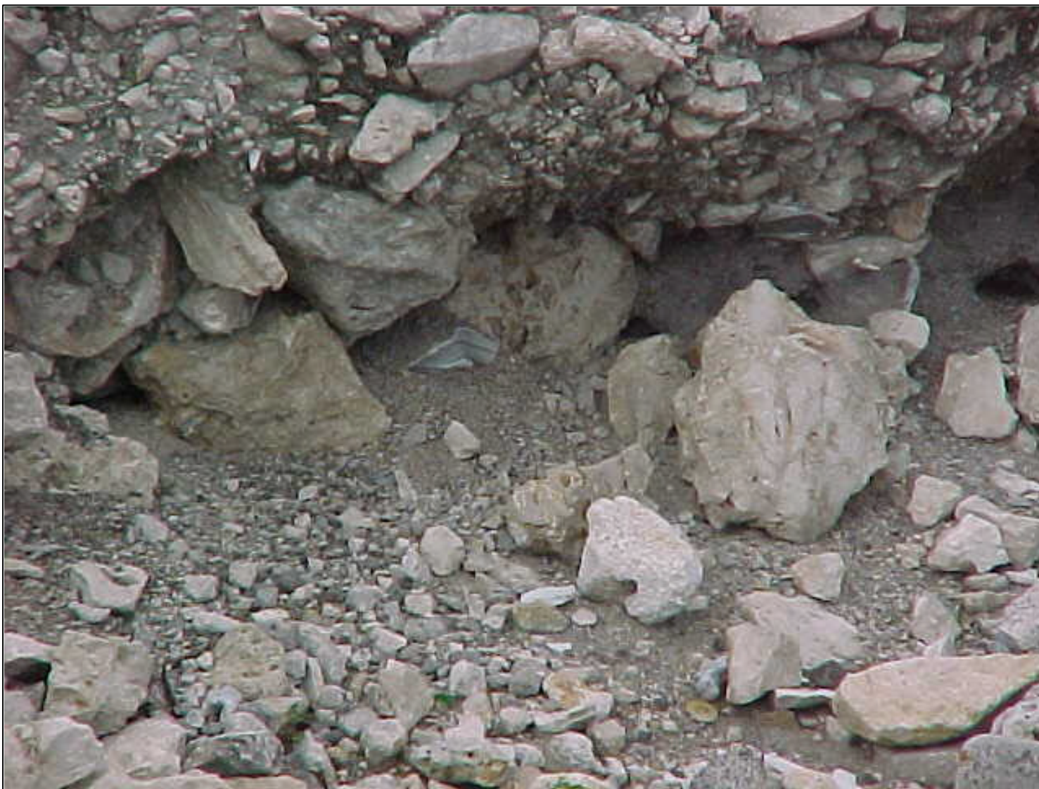
Figure 25. Characteristics of the scoured area at the erosion scarp in Figures 23 and 24. Note the exposed aggregate fill.
