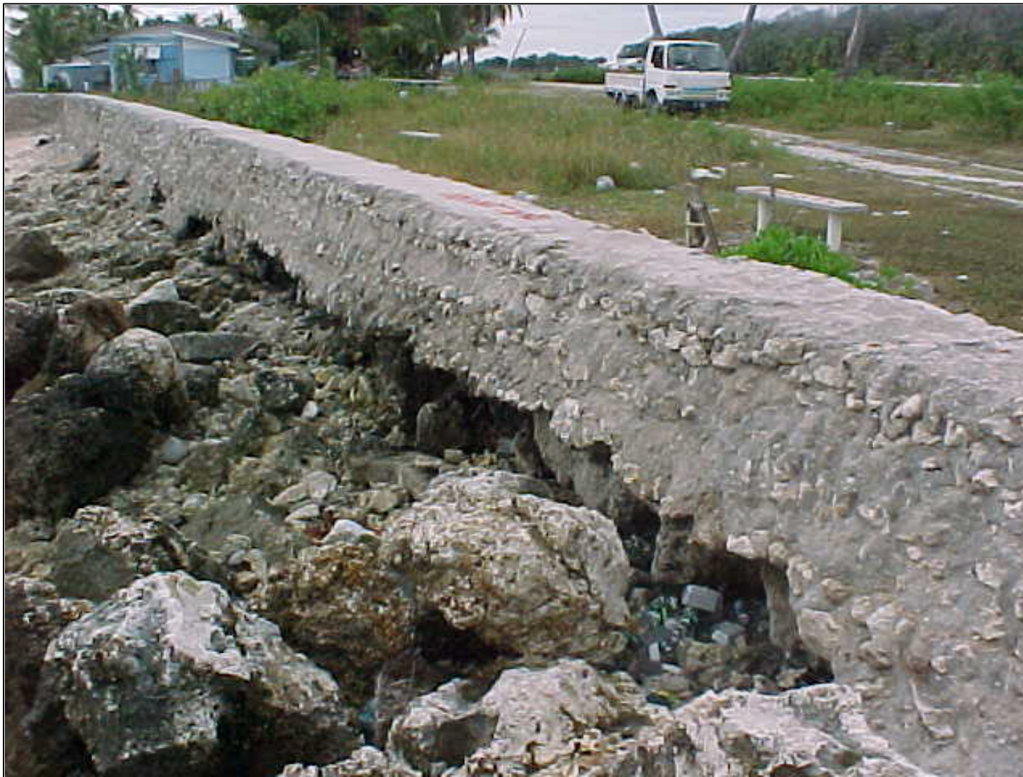
Figure 18. Basal scouring of the retaining wall in Figure 16.
