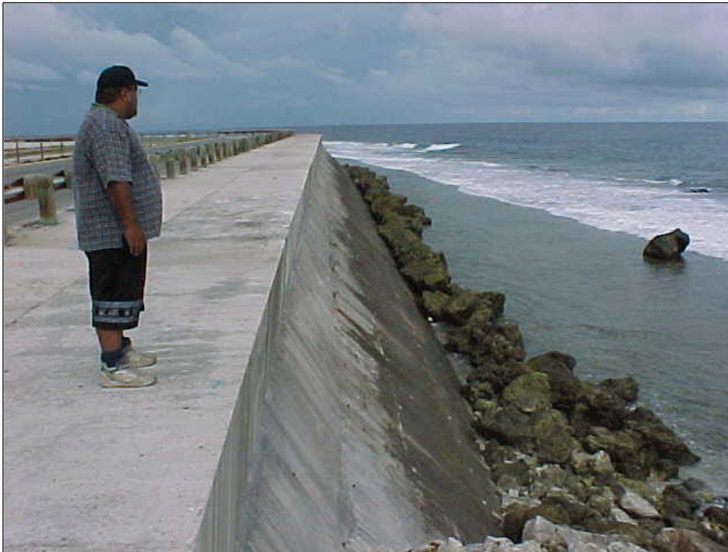
Figure 26. Gravity concrete retaining wall at the outer perimeter of the airport fill site. Looking east.
