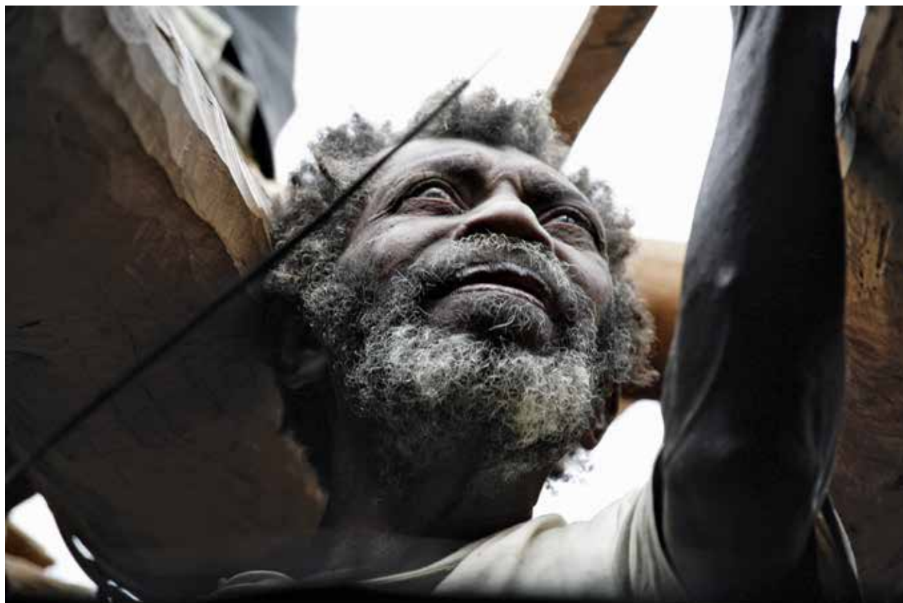
Figure 122: ni-Vanuatu replacing a thatched roof on the chief's meeting hall. (Rob Maccoll/AusAID CC-BY-2.0)
