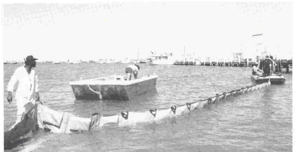
Deployment of shoreline and harbour booms.
