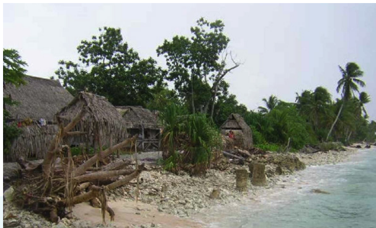
Coastal erosion threatening village.
