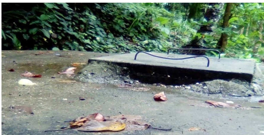
A ferro-cement water storage used by the local communities. Project officers along with zone representatives, conduct physical checks on community water sources and storage. All information feeds into the risk and hazard identification process and feedback from zone representatives to households. Image credit: Water for Women, Solomon Islands
