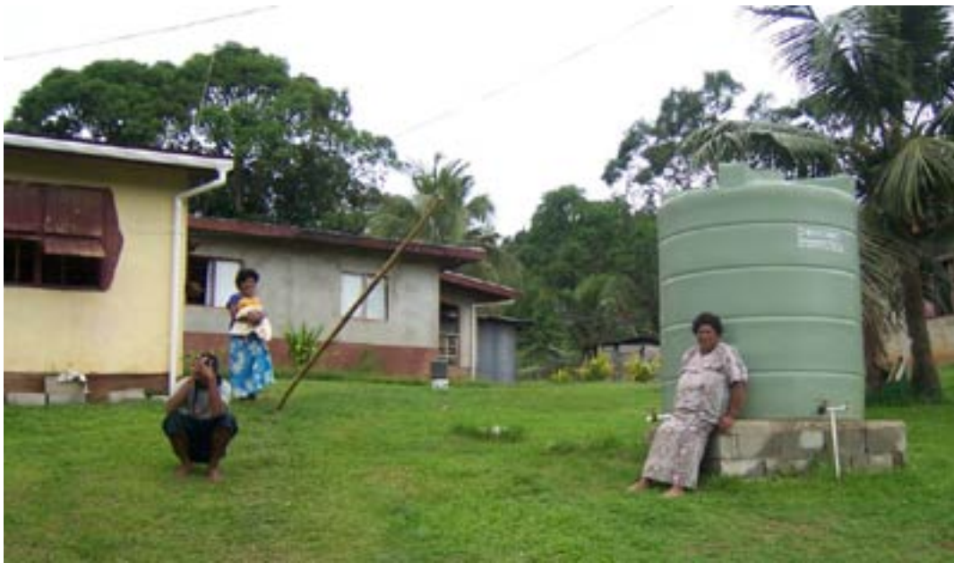
New roof-fed communal water tanks at Bavu
